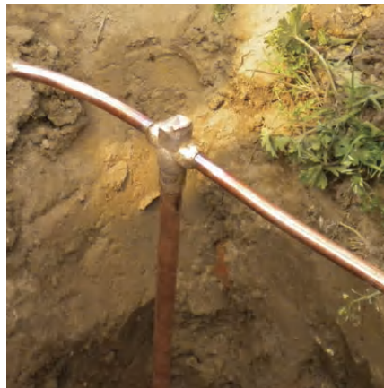
GT Cadweld connection
