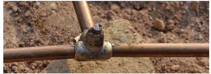
TA nVent ERICO Cadweld connection
